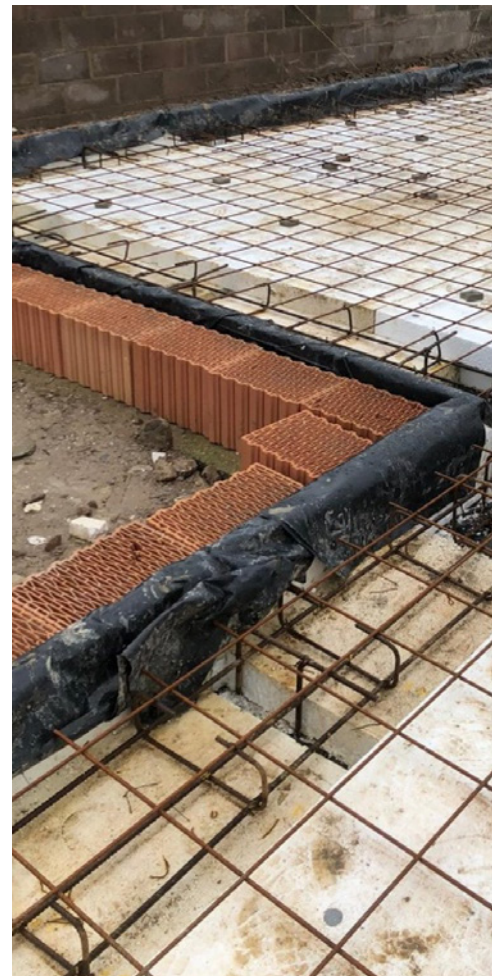
Rebar and Mesh Placed
