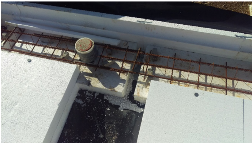
Rebar and Mesh Placed
